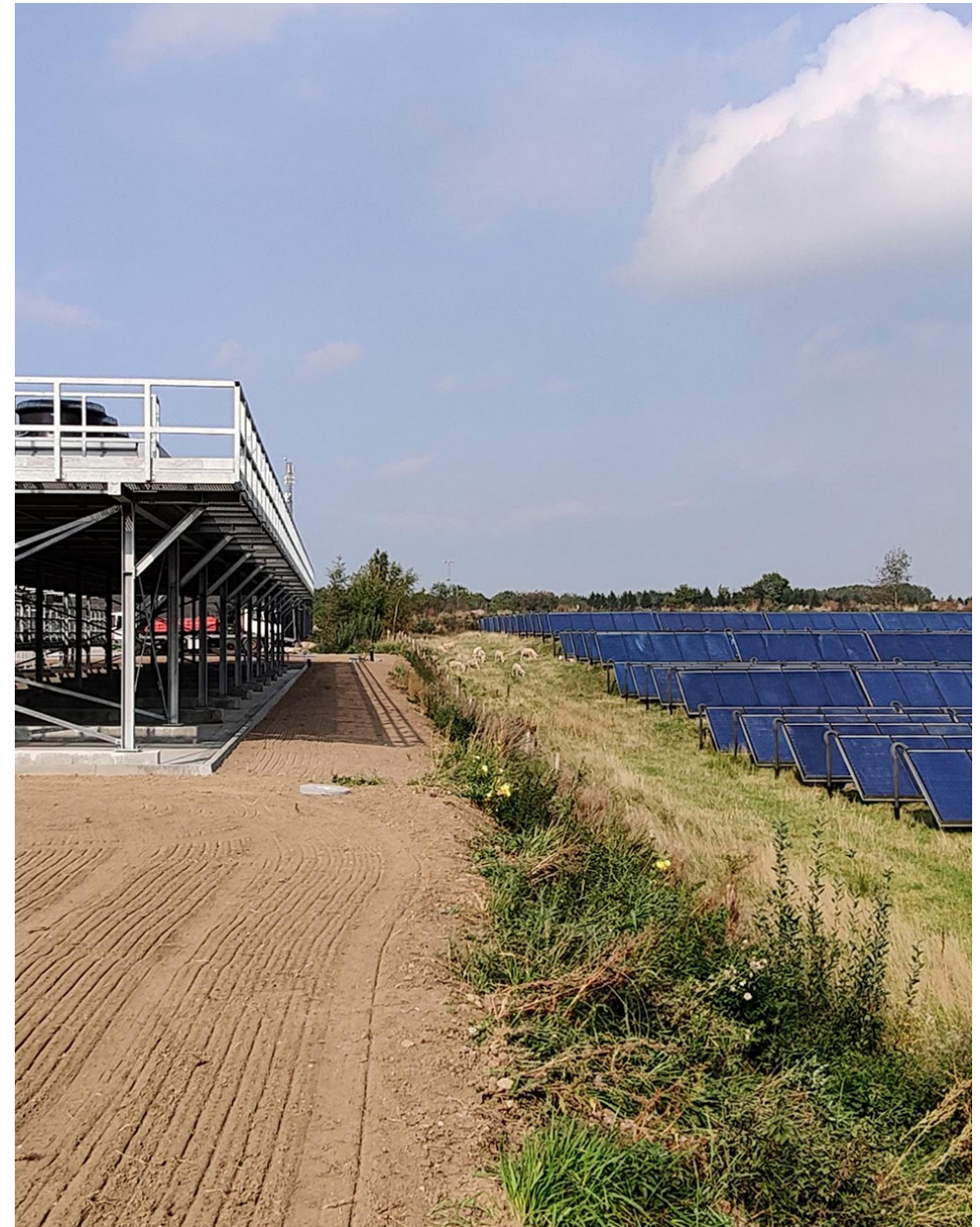
Brædstrup district heating plant to whom Frontmatec has supplied control and S2 SCADA for efficient operation of this state-of-the-art green energy plant.
